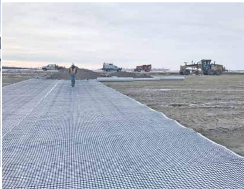
Above: Site development project using TE-BXC geogrid for soil reinforcement.
