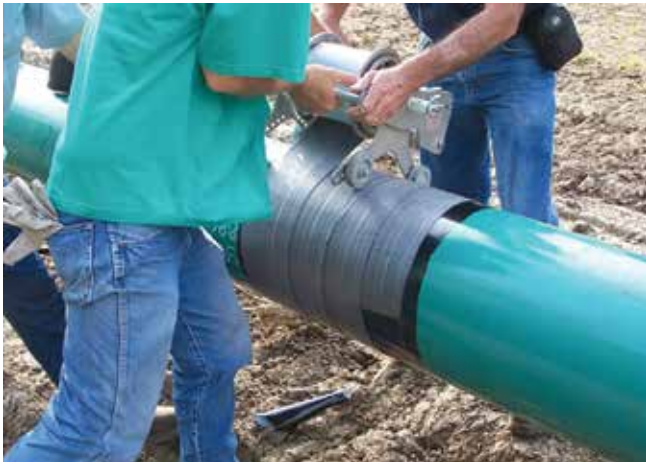
Application of Polyguard RD-6 with wrapster.
