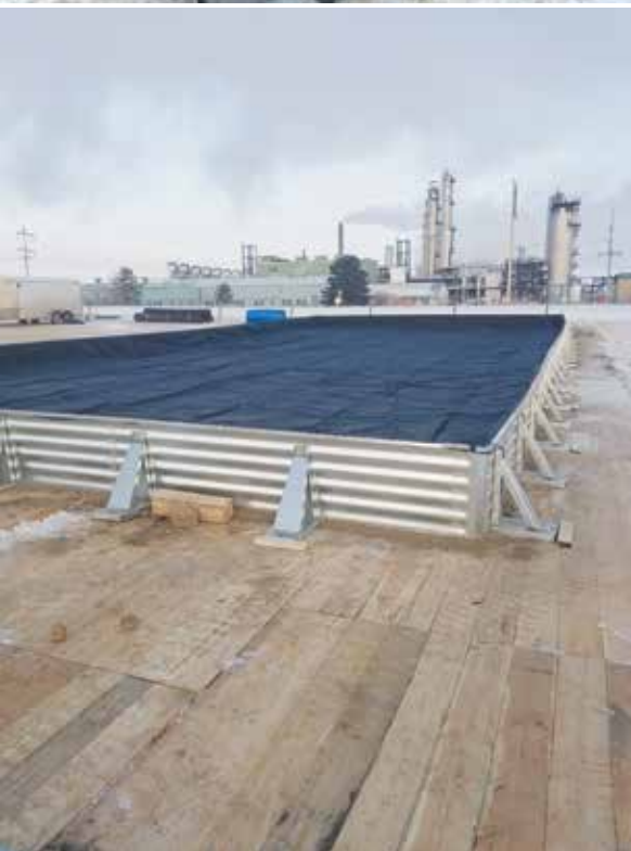
Left: Geomembrane-lined secondary containment system for crude oil storage facility.
