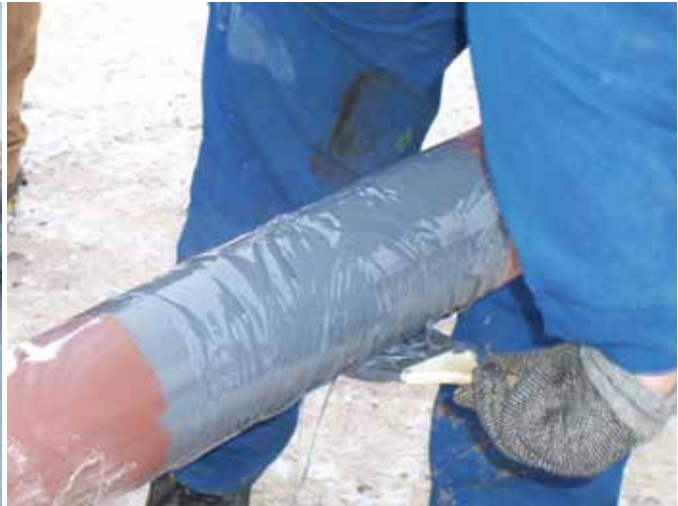
Applying two-part epoxy in cold-weather environment.
