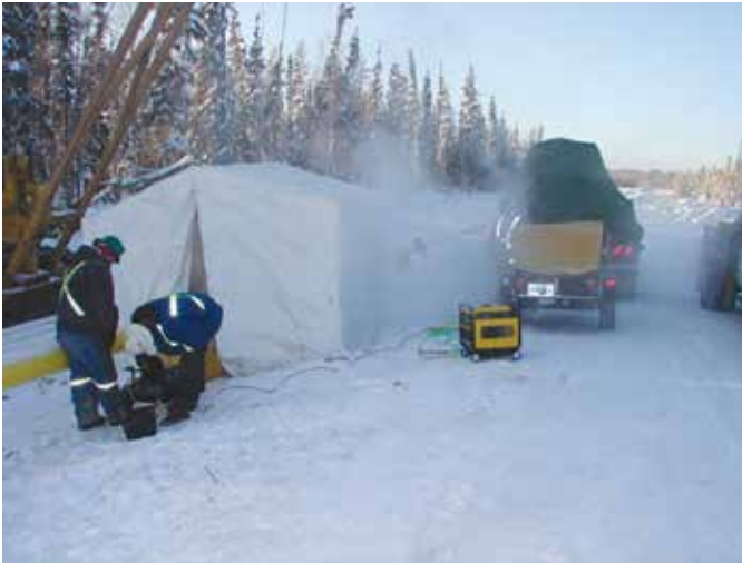
Heated tent in cold-environment coating applications.
